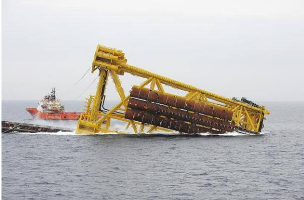
21.05.2013 **The giant Eldfisk II project has taken important steps toward the planned start-up in the winter of 2014/2015. The jacket for the new platform – Eldfisk 2/7 S – is now in place on the field, while construction of the topsides is on schedule on Stord.**
